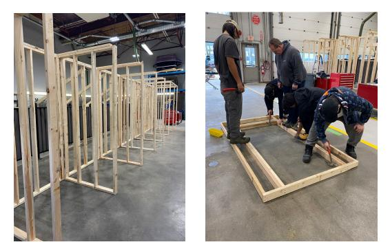
In carpentry, students were given the task of building a 40-foot-long wall out of 2 x 4s using hammers and nails. In the construction process, students were instructed on how to follow specific instructions from a drawing and given measurements to build the structure. Once the students completed the wall structure, they divided the wall into 5-foot cubical sections, which each student would be responsible for.
